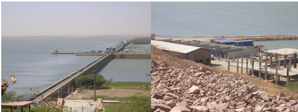
White Nile at JAWN river crossing (l), Jebel Aulia water treatment plant (r)
